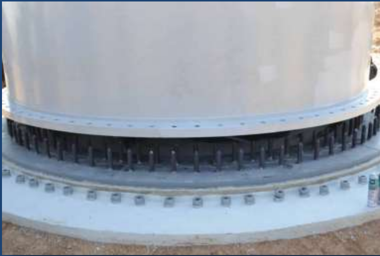
Bottom Section Installation
