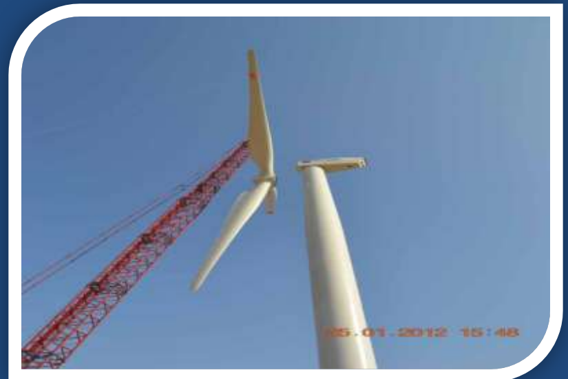
Rotor Hub being Installed
