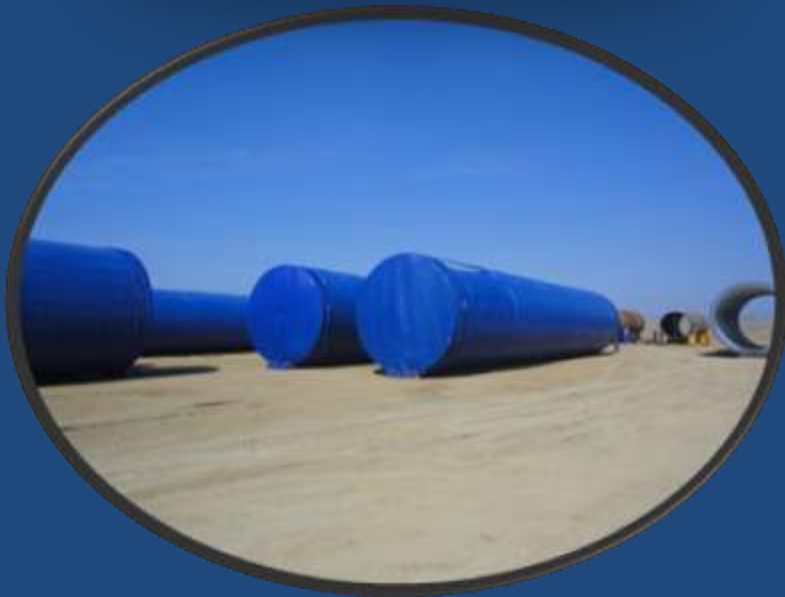
Storage of Sections After Painting
