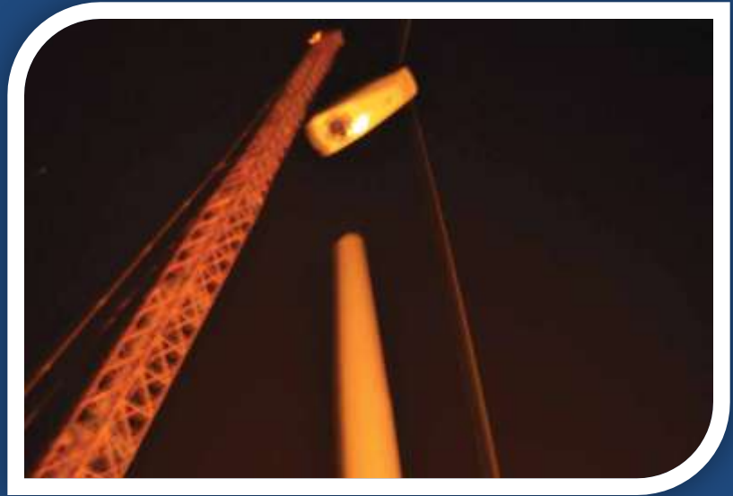
Nacelle being lifted
